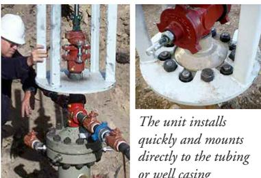
The unit installs quickly and mounts directly to the tubing or well casing
